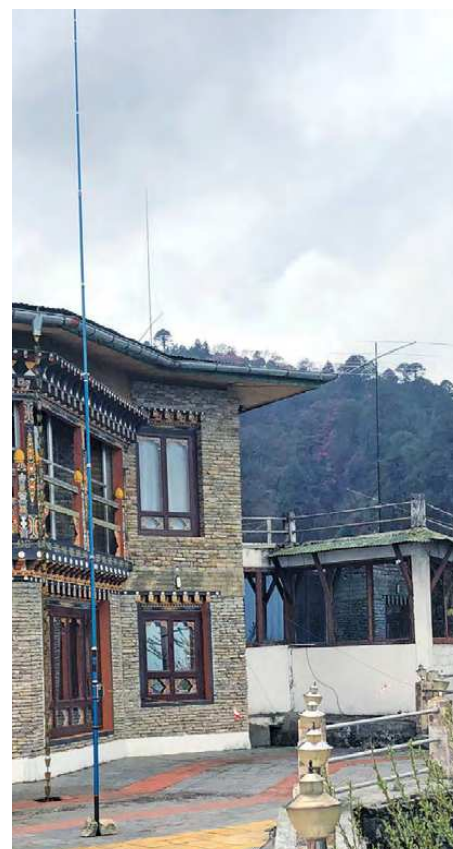
Antennas set up at the Dochula Eco Retreat hotel, 3,150 meters above sea level. [Janusz Wegrzyn, SP9FIH, photo]
